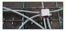
Floor/Ceiling Assemblies Kwikon's light weight and versatility make it perfect for slab applications. Integrated with our slab boxes.
